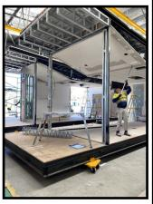
fit out begins. Insulation, electrical works, cabinetry fit outs and underfloor plumbing all take place at the factory before the modules are transported to their new home. We expect to see the first modules arrive in Term 4 for our Performing Arts building and the modules for our new library should arrive later in the term.
